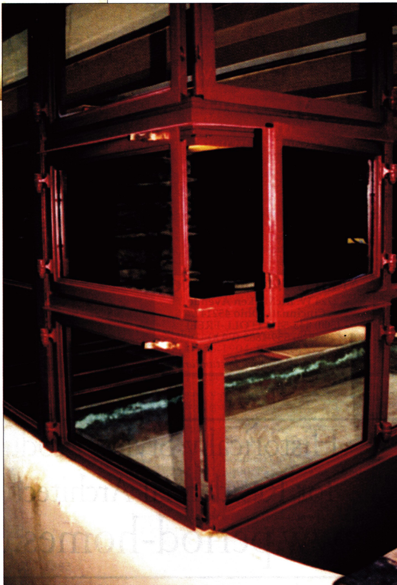
Once restored, the hatch windows open and close as designed. Note the brass hardware, which was removed for cleaning, polished to its original glow, and re-installed.
