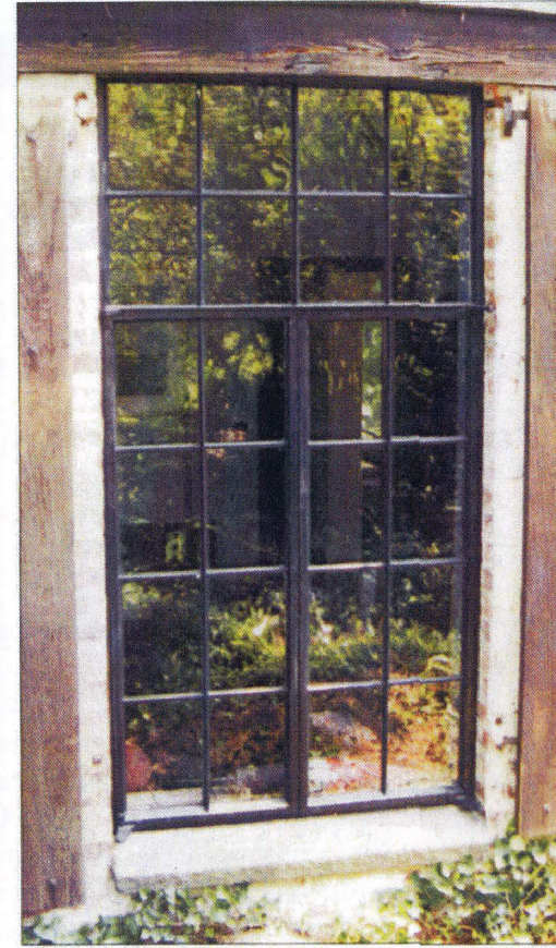
Even though the window in the study was exceptionally large (37 in. wide x 73 in. tall), the Seekirchers were able to find a vintage model (right) with a transom at the top that fit the space. On the left is the worn-out aluminum window.
