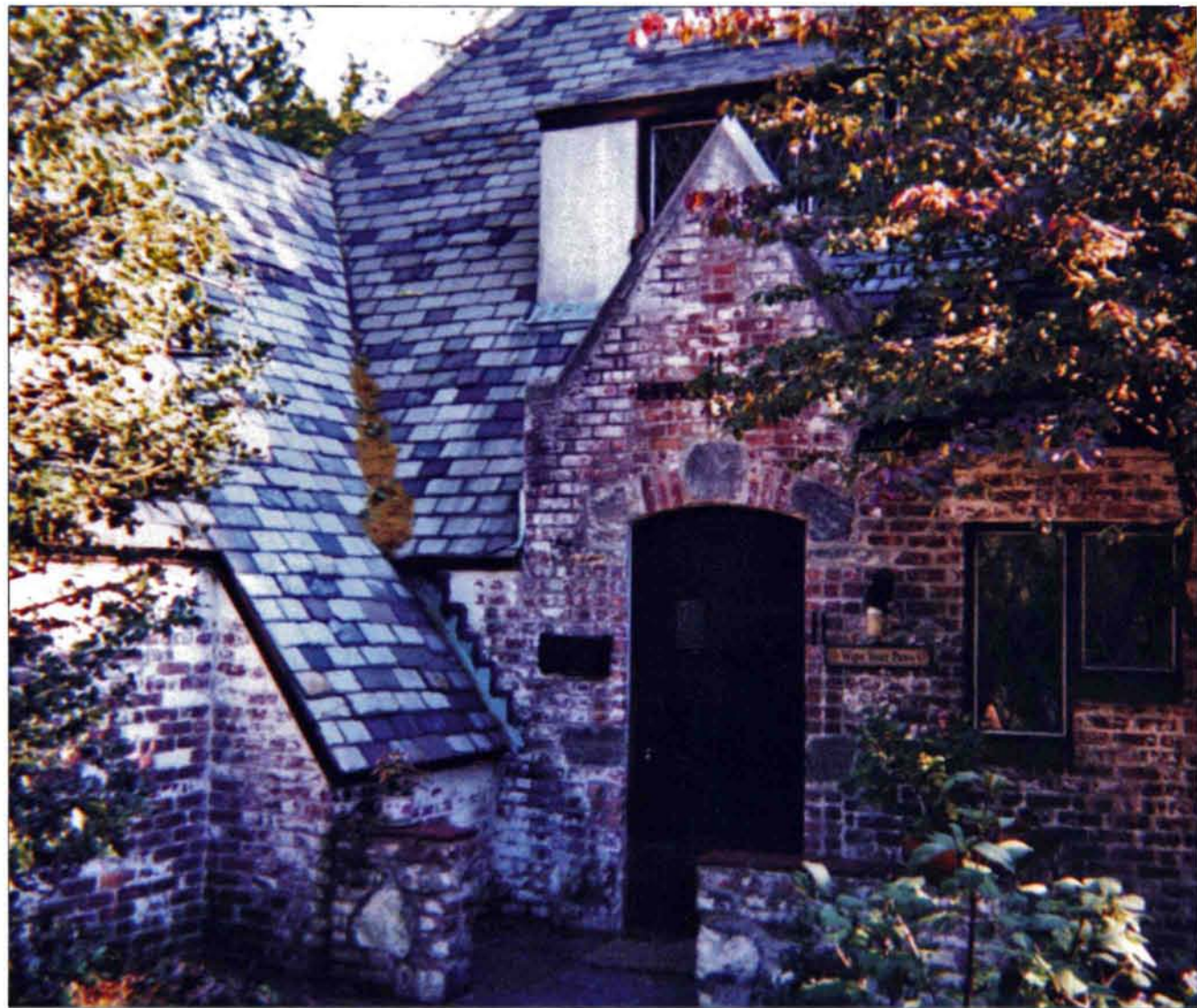
This small Tudor house in Hastings-on-Hudson, NY, regained its charm when the owners replaced the no-longer-functioning aluminum replacement windows with 75-year-old steel casement windows that were supplied and refurbished by Seekircher Window Repair Corp.
