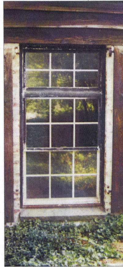
Even though the window in the study was exceptionally large (37 in. wide x 73 in. tall), the Seekirchers were able to find a vintage model (right) with a transom at the top that fit the space. On the left is the worn-out aluminum window.
