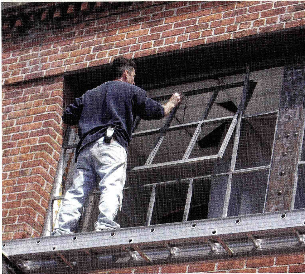
Some of the windows were operational and required only replacement ¼-in. laminated glass, stripping and painting; others were permanently open.
