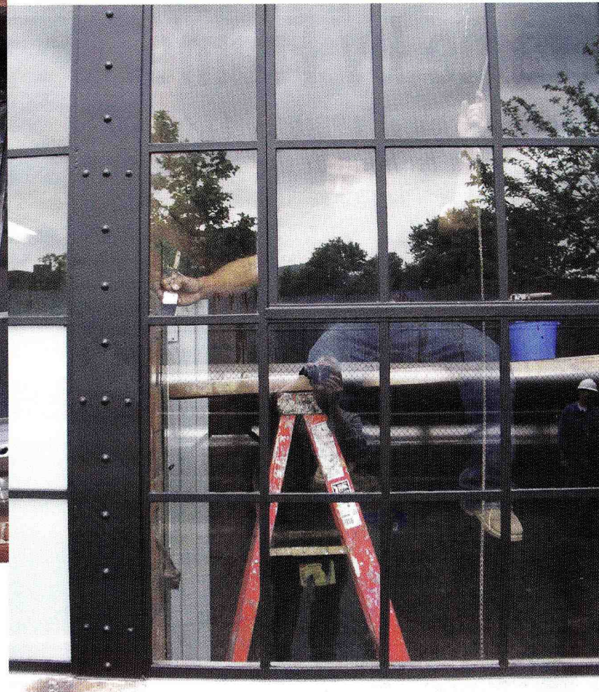
Some of the windows were operational and required only replacement ¼-in. laminated glass, stripping and painting; others were permanently open.
