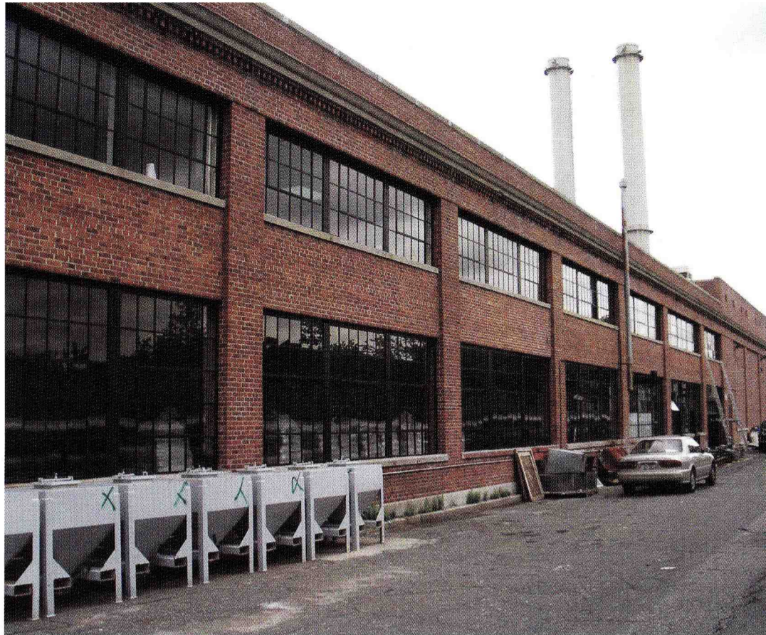
Seekircher Steel Window Repair Corp. restored these original 1920s steel windows at the Brooklyn Navy Yard, making the building an attraction on the Brooklyn Navy Yard Development Corporation's tour of businesses. All photos: courtesy of Walter Sedovic Architects
